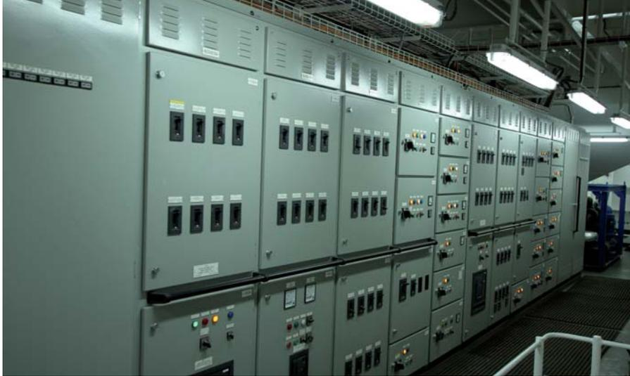
by Ingeteam Marine, regulates engine room equipment and functions. The automatism that carry out this task control 4,000 digital and analogue inputs/outputs.
